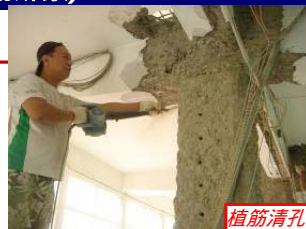
柱梁接頭植筋鑽孔
